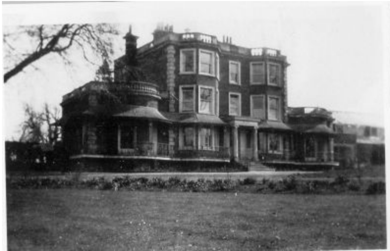
Sackett's Hill House. (Source: Nick Smyth)
